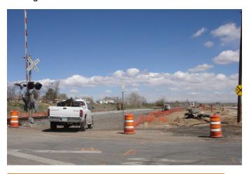
Highway projects involving work on or near railroad tracks or crossings may, in addition to necessary traffic control measures for at-grade crossings, also require the use of railroad flaggers.
