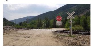
The railroad is responsible for installing and maintaining all crossbuck signs and yield or stop signs, as applicable, at grade crossings.
