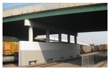
For Highway Underpass Structures, horizontal clearances vary depending on the railroad, curvature of track, future tracks, access roads, and other issues that need to be investigated with the railroads before beginning design. Design must also meet PUC minimum requirements.
